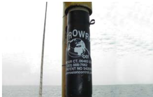
Retrowrap HD dual diameter top seal installed over cut back neoprene reducing down to riser OD. Note rigging lugs for easy rope access installation.
