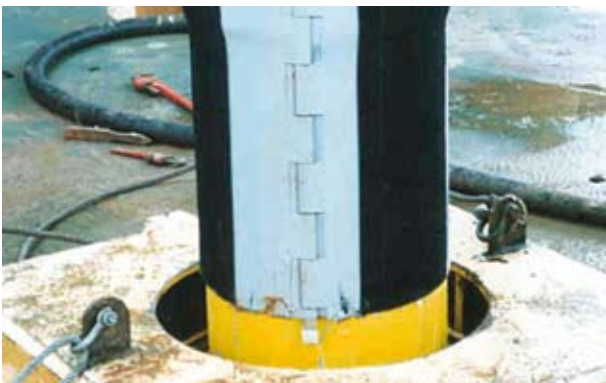
Retrowrap SL installed over Vetco SR 20 conductor connector, Irish Sea.
