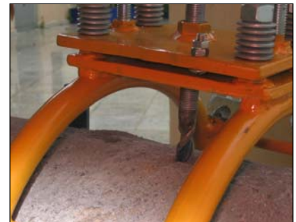
Installed through a concrete weight coat.
