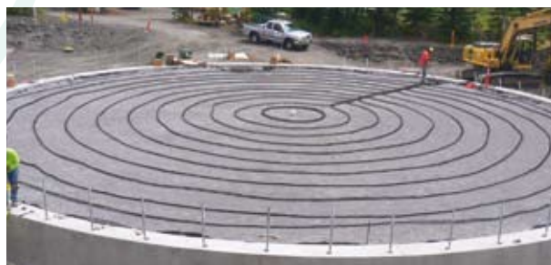
Example of loop system Image courtesy of Ceranode
